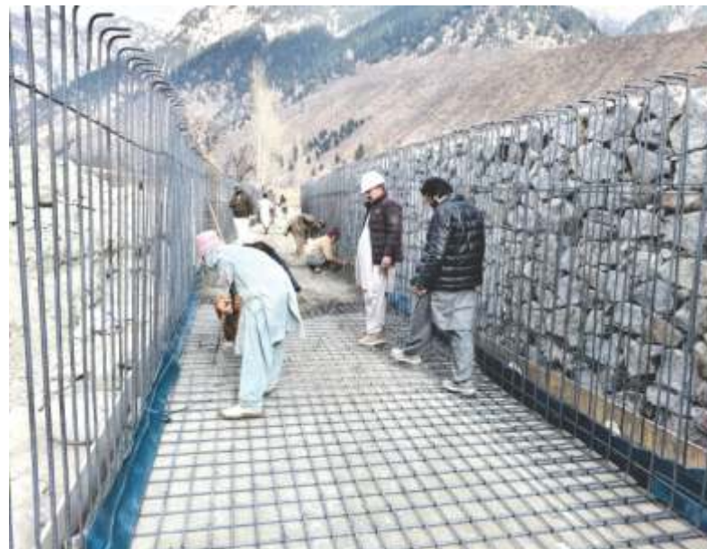
Civil work Thall Kumrat MHP in progress
