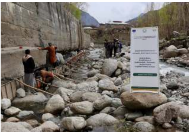
Rehabilitation/Construction of Community Based Irrigation Systems, Darkhanandeh, Lower Chitral
