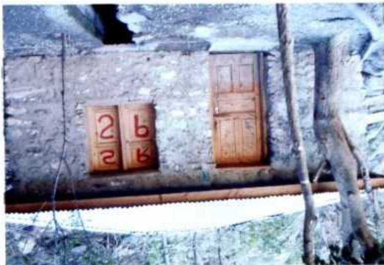
Outside view of power house
