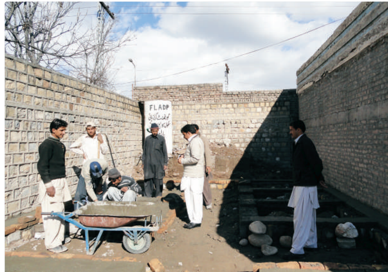
➔ Rehabilitation of a public school for girls in Kurram Agency
